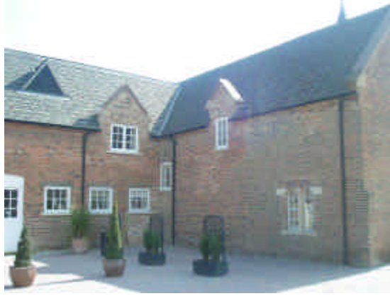
7. Dormer windows subtly added in the style of those existing and other openings formed or closed to suit
