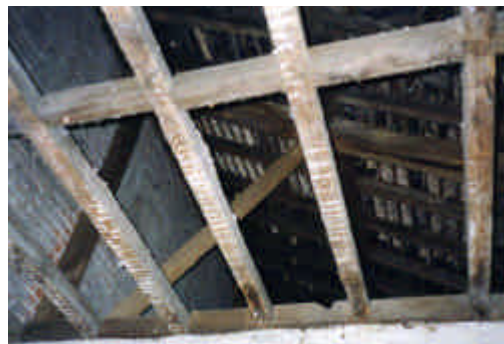
18. The whole roof structure underwent a programme of full restoration and repair
