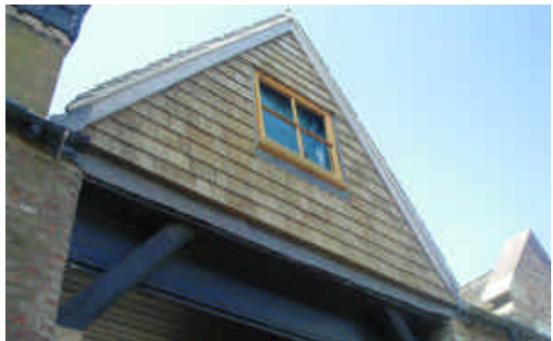
9. New windows, re-clad and re-roofed with timbers restored to match existing
